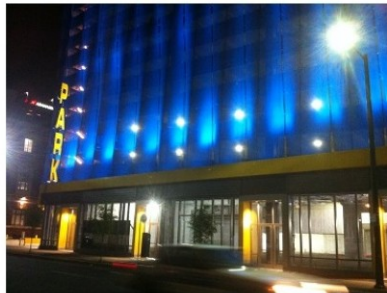
*ACTUAL PICTURE OF PARKING GARAGE*
